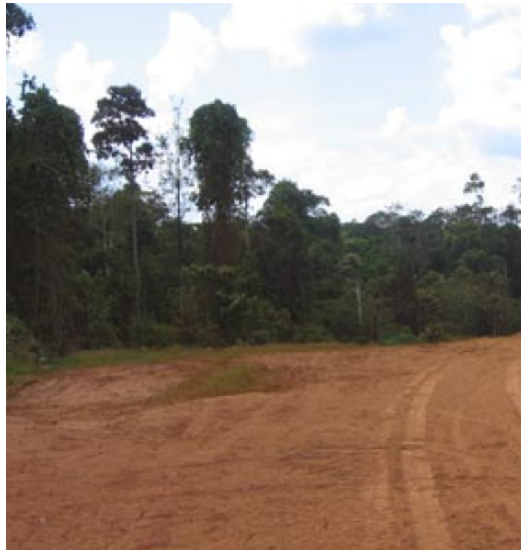
Cleared log road
